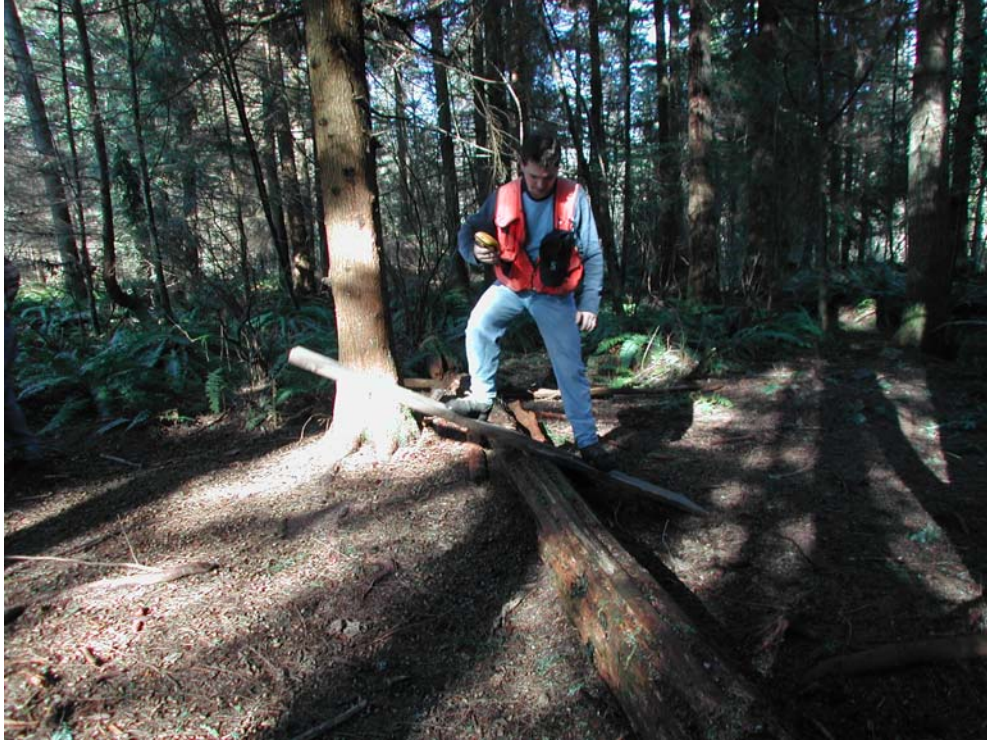
A bicycle “teeter-totter” hinged to a log on the Lloyd Double Diamond Trail
